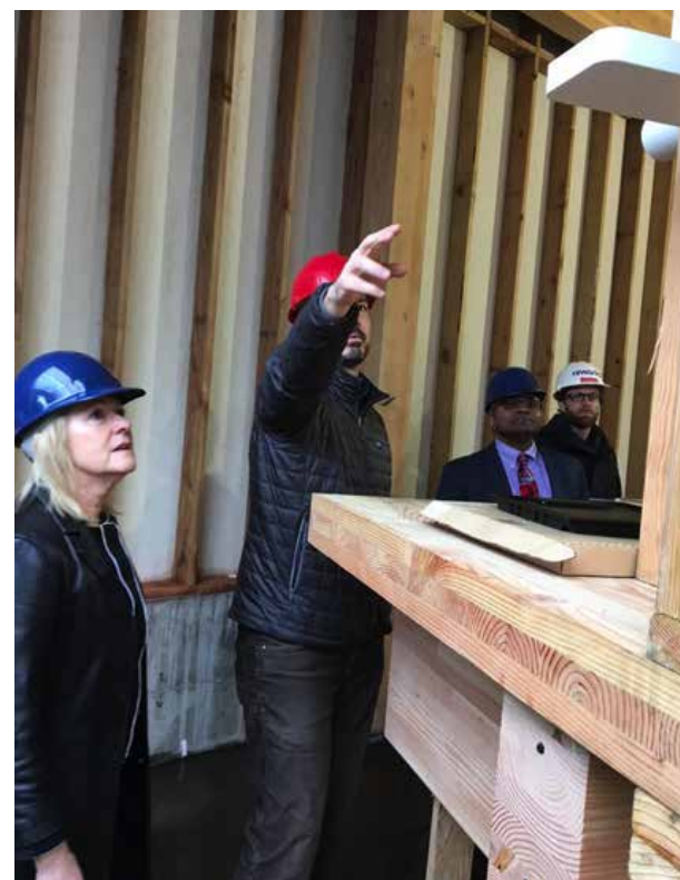
Mayor Lundberg touring the first CLT building in Portland.
